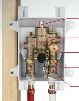
Temperature adjustment stem is 3/8" hex. All valves are tested and preset to  $105^{\circ}$  F
