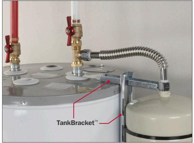
Tee adapters make connecting expansion tanks fast and easy. The TankBracket™ (598-023 shown) supports units directly on heater.
